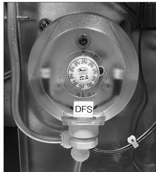
Figure 26.3 - Dirty Filter Pressure Switch
