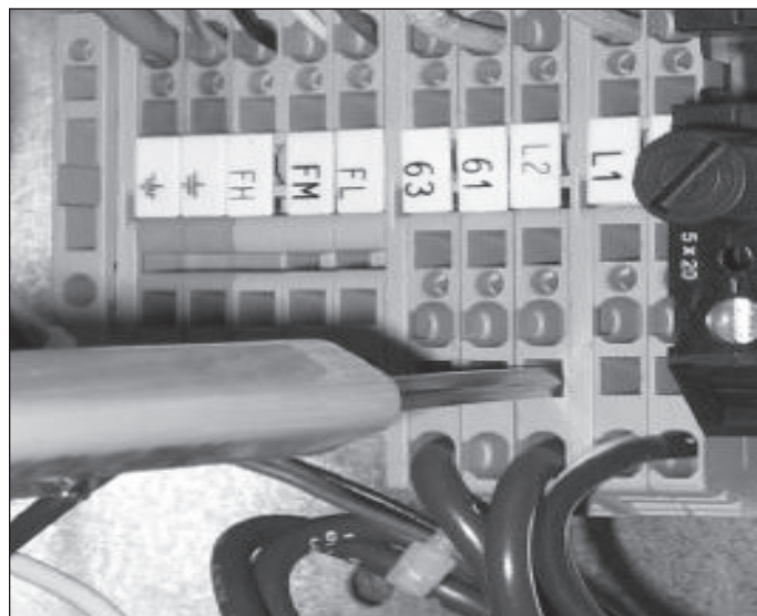
Figure 9.1 - Terminal Strip
