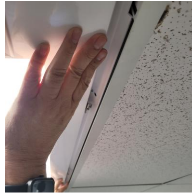
Figure 19: Lock bar will spring out to rest on ceiling frame.
