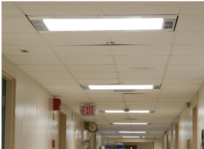
Figure 20: Completed Drop Ceiling Installation
