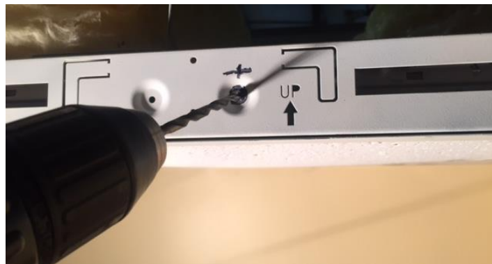
Figure 6: Drilling the Mounting Bracket
