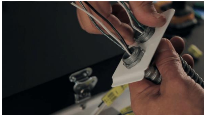
Figure 14: Installing the Wiring Conduit Access Plate
