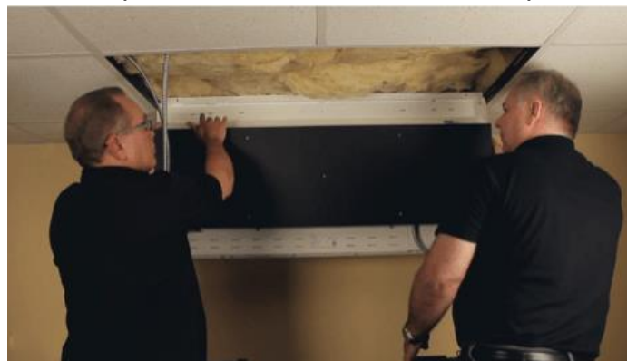
Figure 12: Preparing to Connect Power
