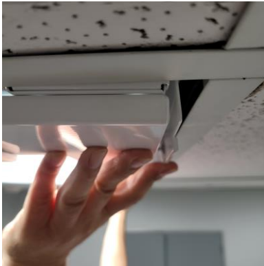
Figure 18: Lock bar pressed flush to unit.
