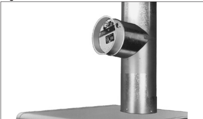
Figure 5.2 - Barometric Draft Control Above Unit
